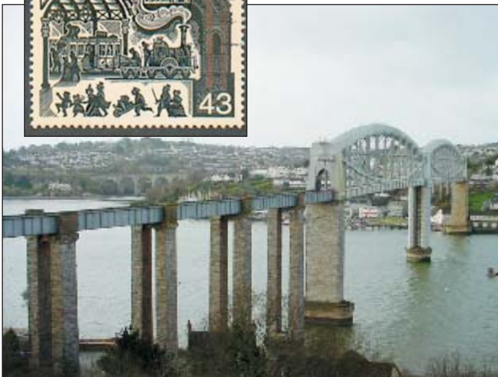
Royal Albert Bridge, Saltash.
